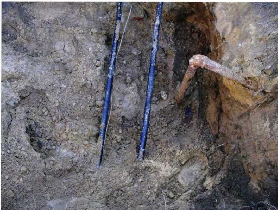
Picture 2: UST 915Barracuda excavation showing vent line and geothermal lines.
